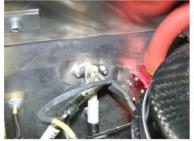
Re-assemble feed through as shown. Torque nut to 30 Nm (266 in-lb) (22 Ft. lbs)
